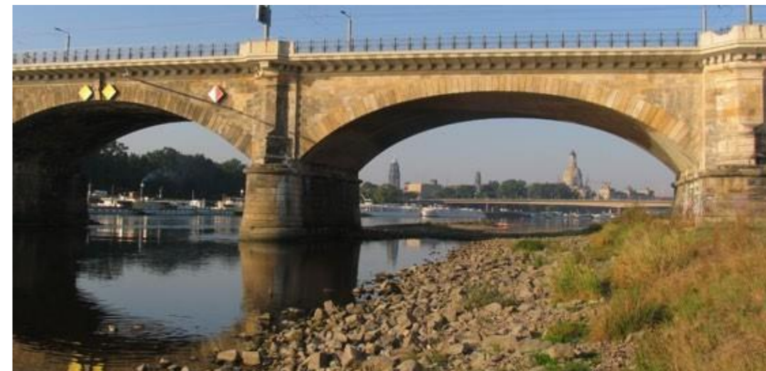
POSTA SANDSTONE, Albert Bridge, Dresden
