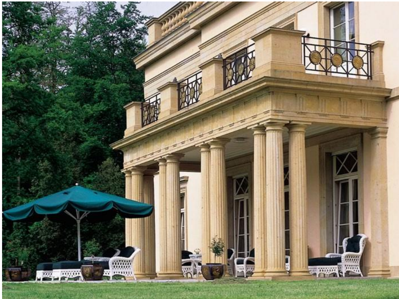
REINHARDTSDORFER SANDSTEIN, private villa, Frankfurt am Main
